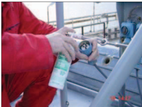
Image 18.b Applying VpCI® 238 for protection of electric contacts
