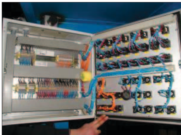
Image 18.a Applying VpCI® Emitter in electric panel
