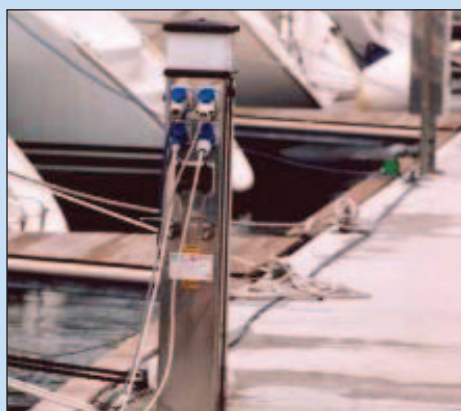
Electrical distribution pedestal
